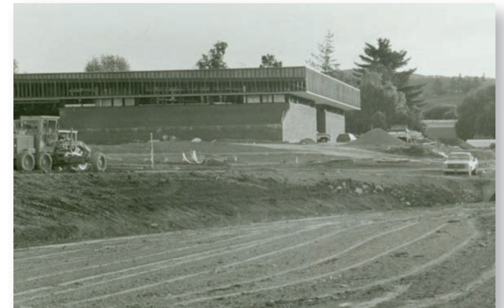
Construction of the Pearson Library and Preus-Brandt Forum in 1984.
