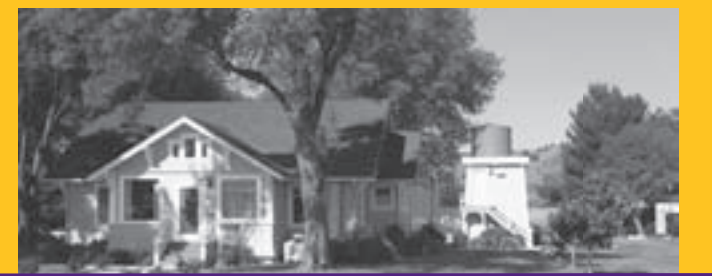
The Pederson ranch house, built in 1913, is a historical landmark.
